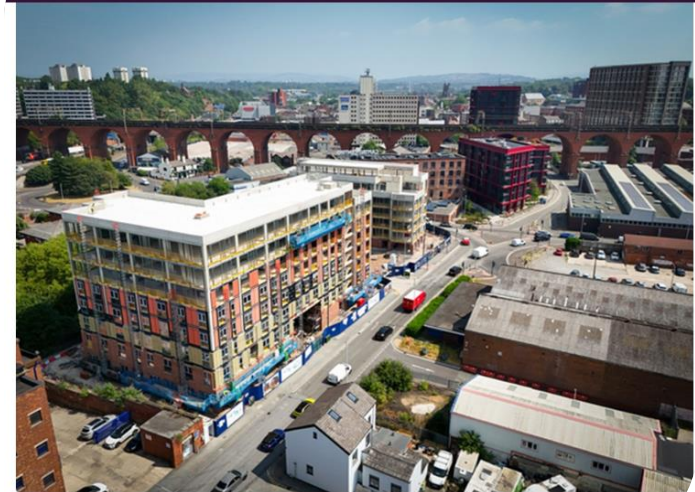
Great Places tops out at Hatters Yard
